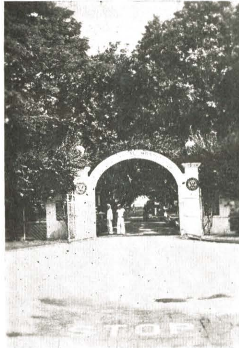
Hospital Main Gate
